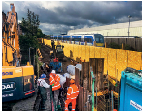
Works Fenced & Segregated from Live Trains: Only permitted with strict controls
