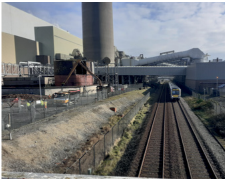
Adjacent Works alongside Live Train: Only permitted with strict controls
