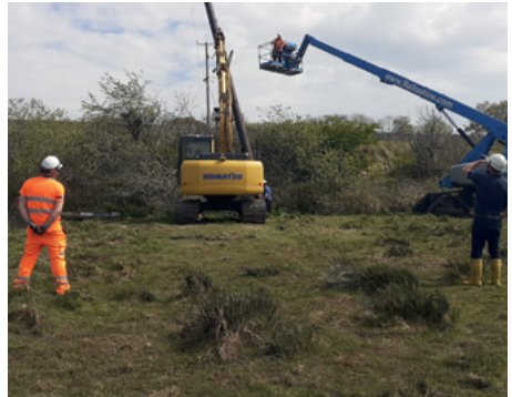
T2 possession: for daytime short duration works between live trains
