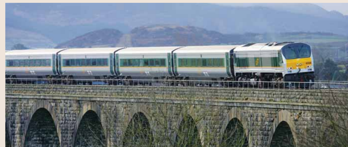
Enterprise train crossing the Craigmore Viaduct at Newry
