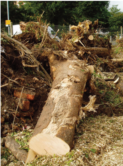
Tree removal on Translink property
