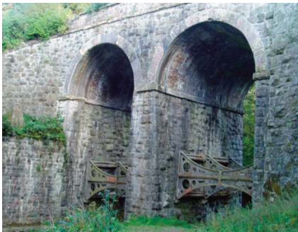
Viaduct at Three Mile Water
